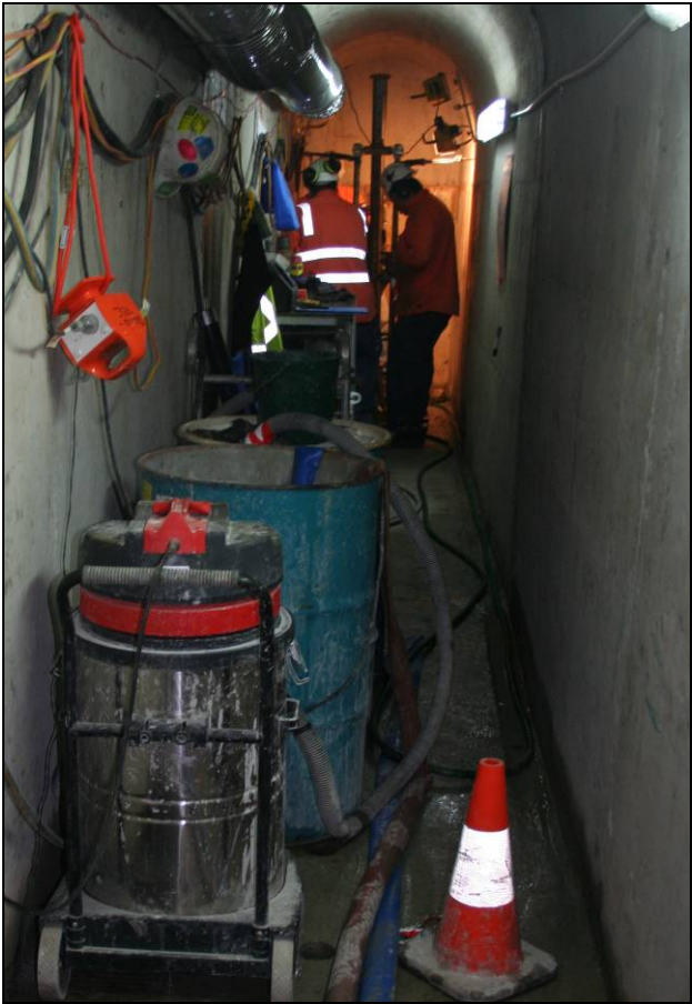
Figure 3 – Left: Gallery Floor Slurry Control System Right: Slurry Collection Tank and Water Supply Tank
