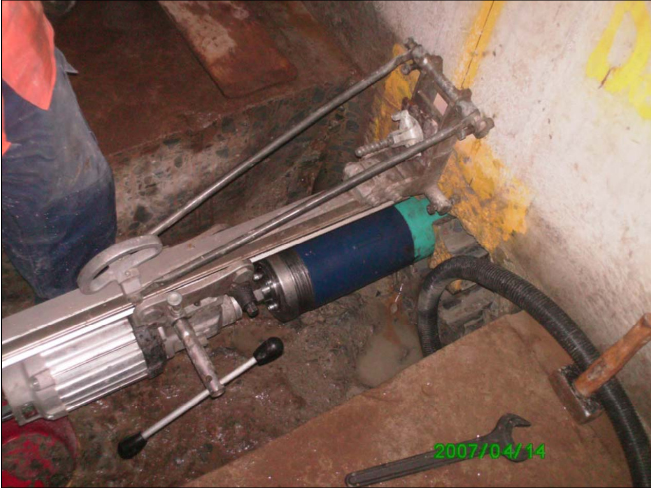
Figure 5 – 160mm Diameter Drain Hole
