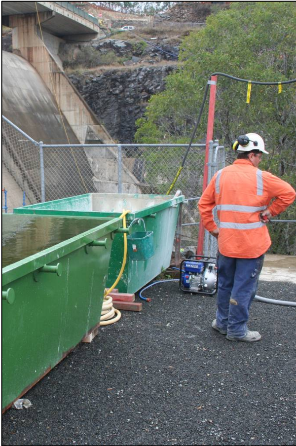
Figure 3 – Left: Gallery Floor Slurry Control System Right: Slurry Collection Tank and Water Supply Tank
