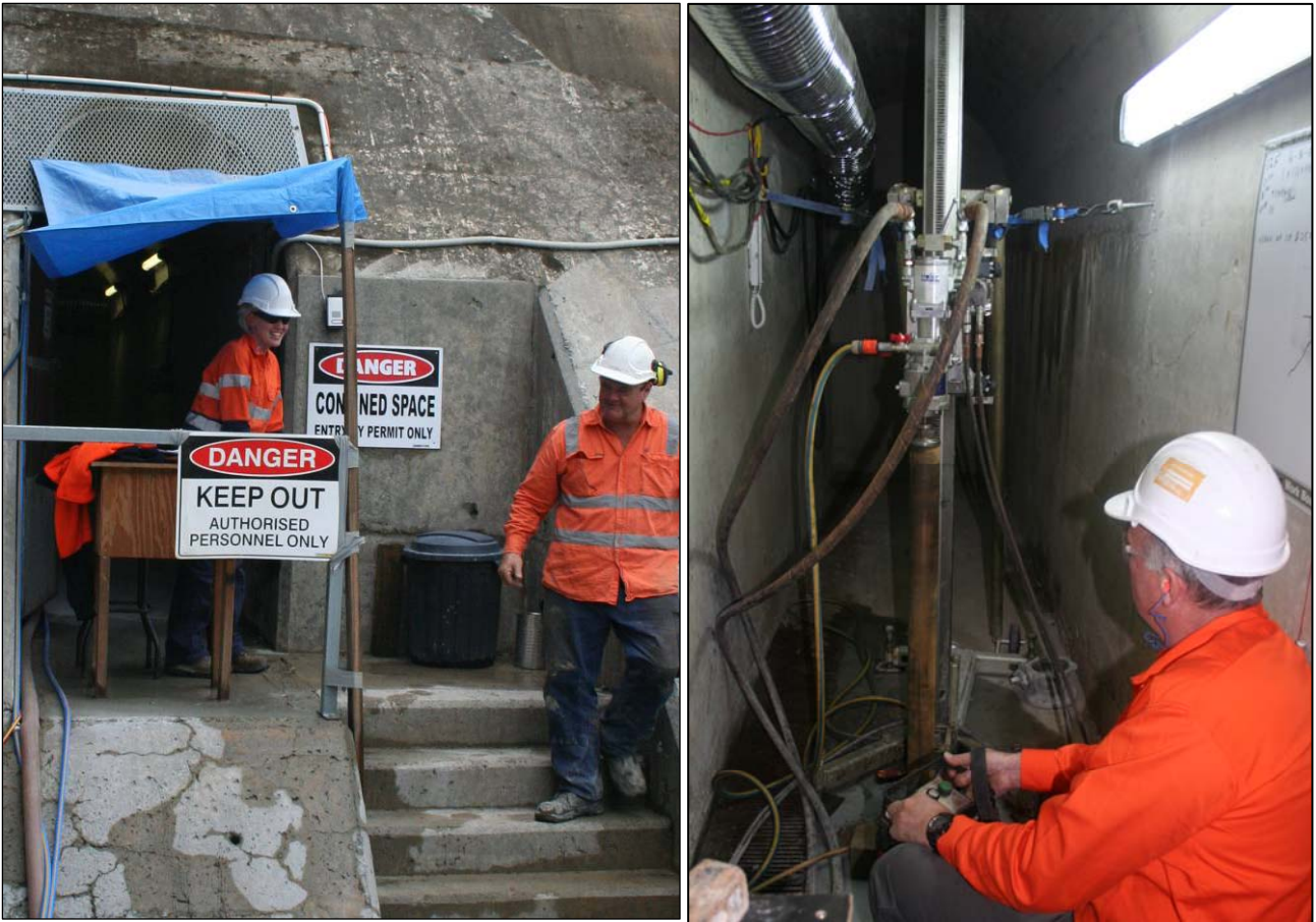
Figure 2 – Left: Entrance to the Spillway Drainage Gallery Right: Hydraulic Drilling Equipment
